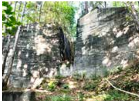
▲ Ruins of Iron Mill near Soleil Clubhouse. (Photo by Brian Paley)
